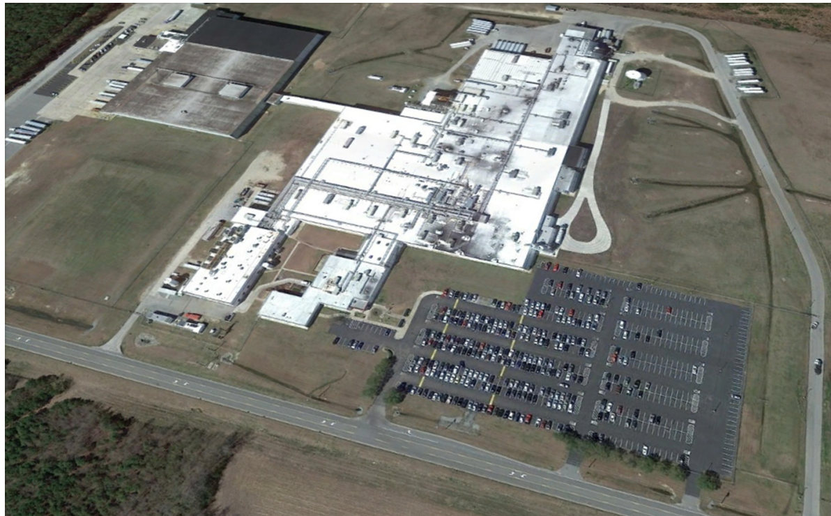
Figure 18: Aerial View of Hillshire (Tyson Foods) wholesale bakery and distribution center.
