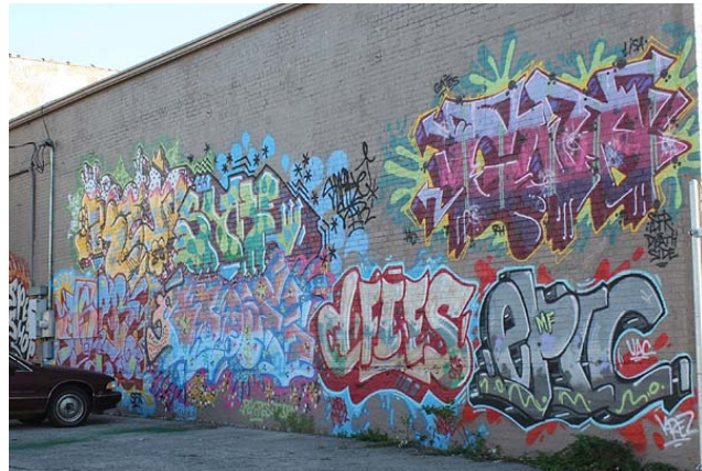
Gang graffiti covers the side of this building.
