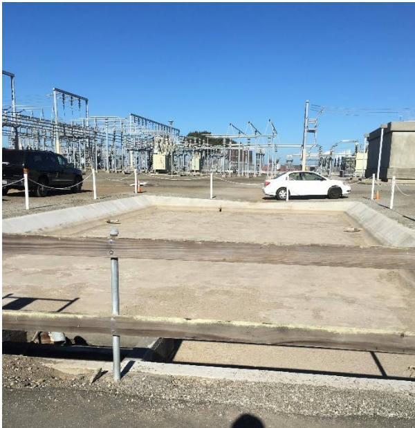
Figure 1: Spill retention pond
